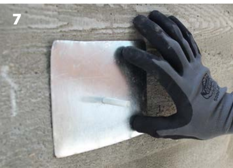
To ensure protection of exposed concrete surface, drill sheet metal 3/8" hole and slide over rod, then cut.
