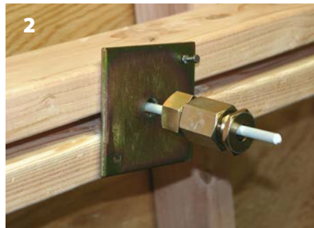
Slip Bearing Plate and Gripper onto the fiberglass rod. For a battered wall, add wedge shaped spacers so that the fiberglass rod is kept straight. The strength of a bent rod is significantly reduced.
