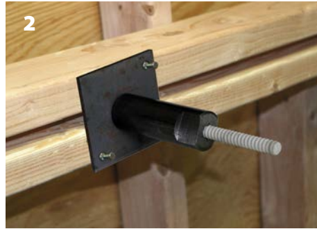
2 Slip Bearing Plate and Form Fixture onto the fiberglass rod. For a battered wall, add wedge shaped spacers so that the fiberglass rod is kept straight. The strength of a bent rod is significantly reduced.
