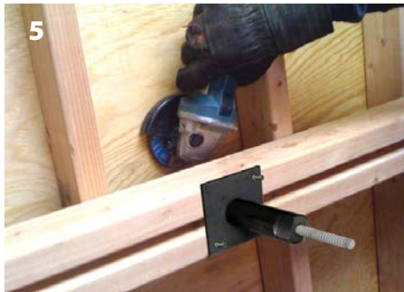
5 Cut the fiberglass rod between the Form Fixture and the form.
