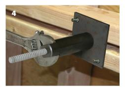
On the opposite side of the form, lock another Form Fixture onto the fiberglass rod.
