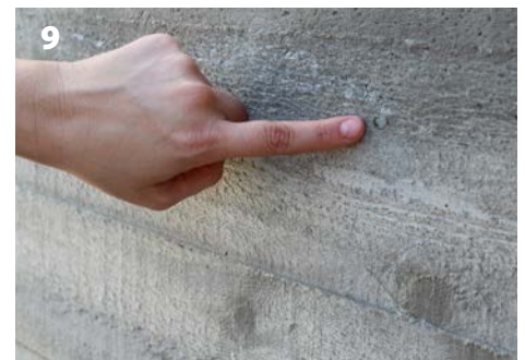
9 The tie will nearly disappear. No breakback. No plugging. No patching.
