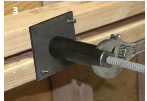
3 Lock the Form Fixture onto the fiberglass rod by turning the "Form Fixture" clockwise.
