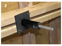
Slip Bearing Plate and Form Fixture onto the fiberglass rod. For a battered wall, add wedge shaped spacers so that the fiberglass rod is kept straight. The strength of a bent rod is significantly reduced.
