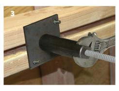
Lock the Form Fixture onto the fiberglass rod by turning the "Form Fixture" clockwise.
