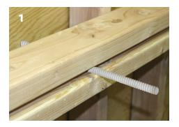
Slide the fiberglass rod through the form. Short lengths of fiberglass rod can be used as internal spreaders; these spreaders can be either tied to the rebar cage, or attached to the tie rod by using two Spreader Clips.
