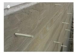
After removing the forms, you will see short lengths of fiberglass rod sticking out of your structure.
