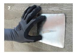
To ensure protection of exposed concrete surface, drill a hole slightly larger than rod diameter in a piece of sheet metal, slide over rod, then cut.
