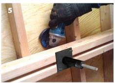
Cut the fiberglass rod between the Form Fixture and the form.
