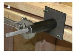
On the opposite side of the form, lock another Form Fixture onto the fiberglass rod.
