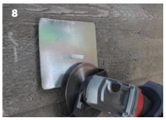
Grind the stubs of fiberglass rod off flush to the concrete structure using a grinder with a diamond blade.
