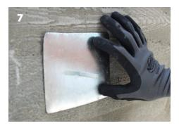
To ensure protection of exposed concrete surface, drill sheet metal 3/8" hole and slide over rod, then cut.
