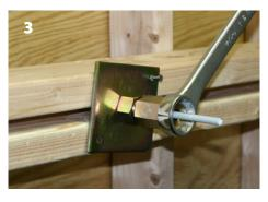
Lock the Gripper onto the fiberglass rod by turning the "tightening bolt" clockwise (min. 15 ft. lbs.) On the opposite side of the form, lock another Gripper onto the fiberglass rod.
