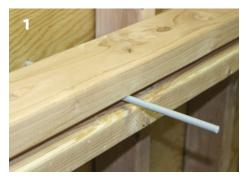
Slide the fiberglass rod through the form. Short lengths of fiberglass rod can be used as internal spreaders; these spreaders can be either tied to the rebar cage, or attached to the tie rod by using two Spreader Clips.
