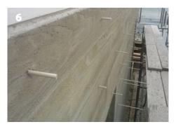
After removing the forms, you will see short lengths of fiberglass rod sticking out of your structure.
