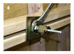
Use the "tensioning nut" to adjust width of form, or tighten form against internal spreaders (there is a maximum of 1/2" of adjustability for each Gripper). You are now ready to place concrete.
