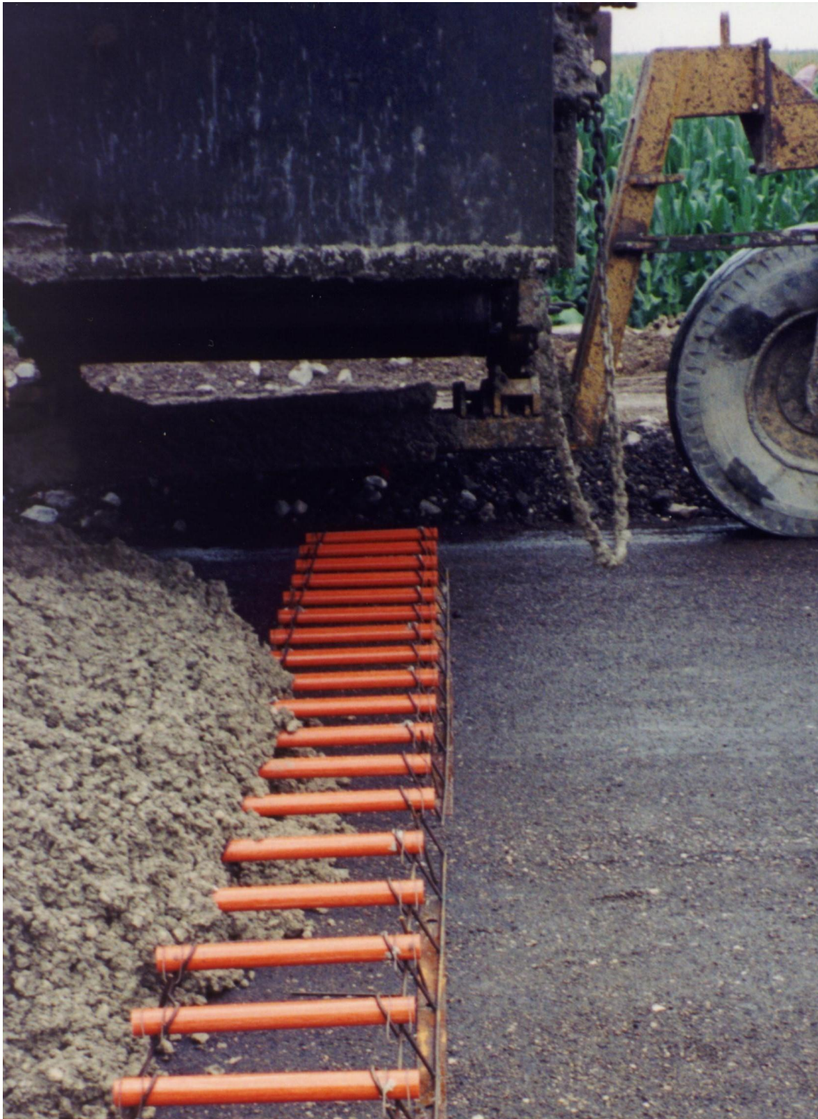
FiberDowel being paved over by IL-DOT (9/97)
