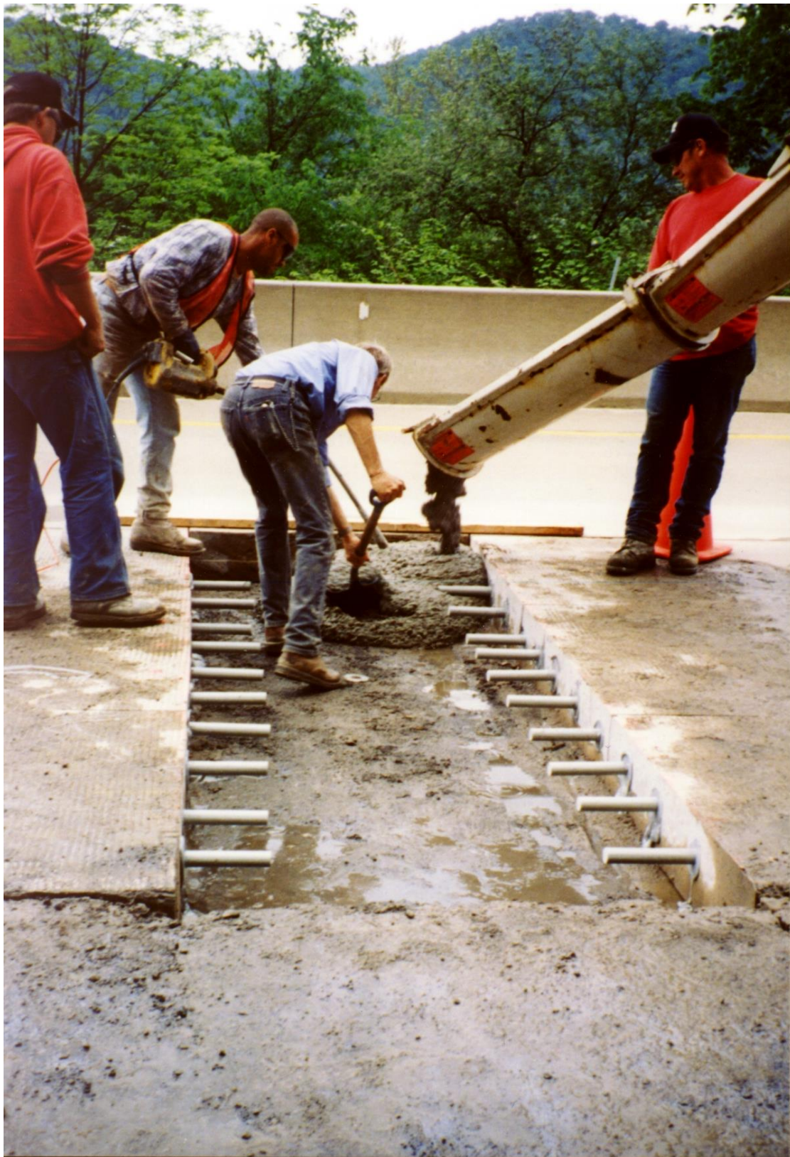
FiberDowel Material Studied after 14 Years in use by O-DOT
