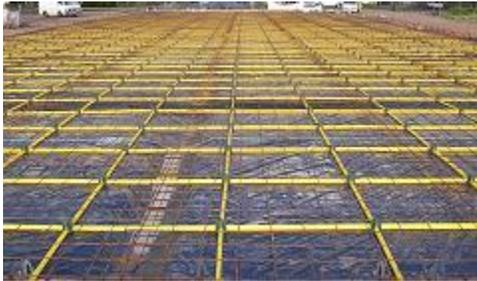
**Joint free slabs** use a plastic grid (*left*) to induce a closely spaced network of fine cracks throughout the entire length and breadth of large-area slabs on grade, and thereby eliminate all traditional formed and sawn shrinkage control joints.
