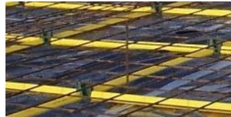
The full perimeter of each **joint free slab** pour is trimmed with 2N12 bars and special attention is paid to the trimming of re-entrant corners and penetrations.
